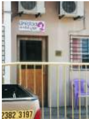
I. Shelter entrance within the Municipal facility
